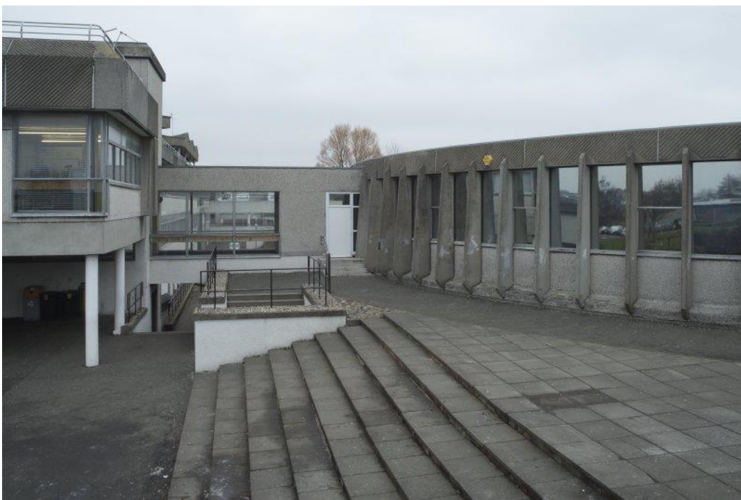
Inverkeithing High School, Fife. 1968-73. Listed category B in 2004.
