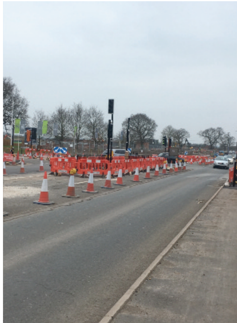
Transport Infrastructure is always a discussion surrounding viability.
