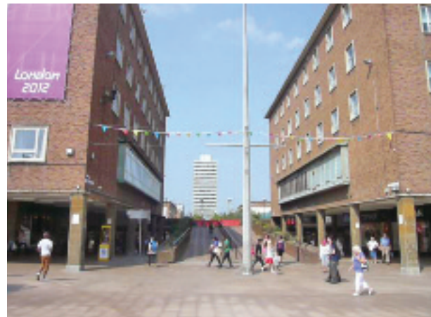
Coventry Upper Precinct, Listed despite intrusive ramp.
