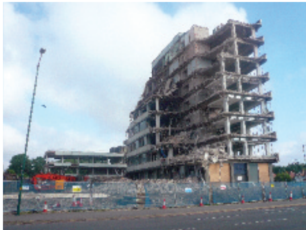
Madin's Powergen (Midlands Electricity Board) building, Shirley, being demolished 2018.
