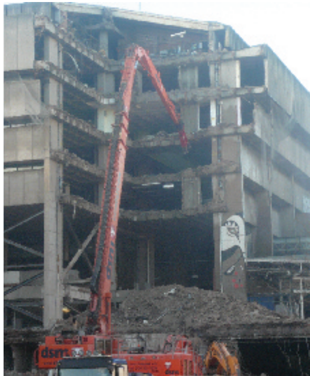
Madin's Birmingham central Library being demolished, 2016.
