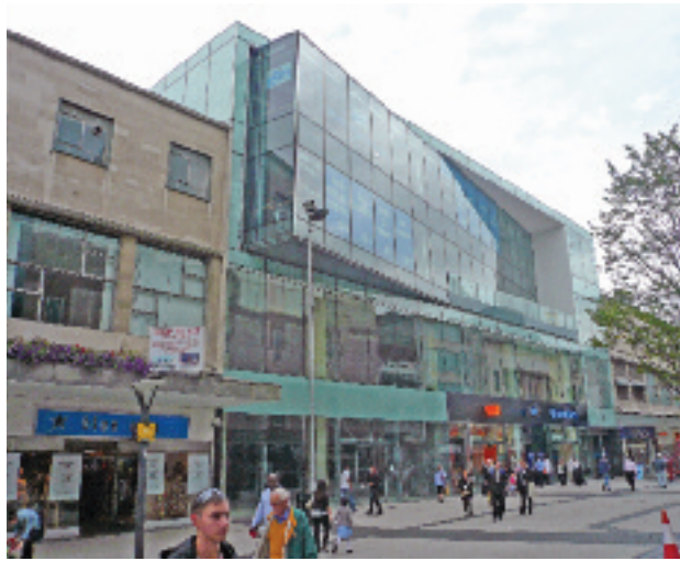
New front, "Big Top" site, High Street Birmingham (the section to the left is now being worked on, both retain the original concrete skeleton).
