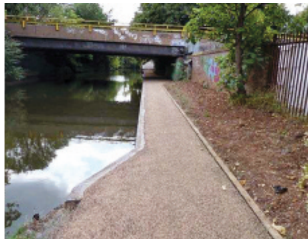
Grand Union Canal, Birmingham, after improvements. Upgraded to bonded surfaces.
