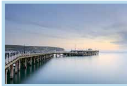
Swanage Pier Restoration & Regeneration
